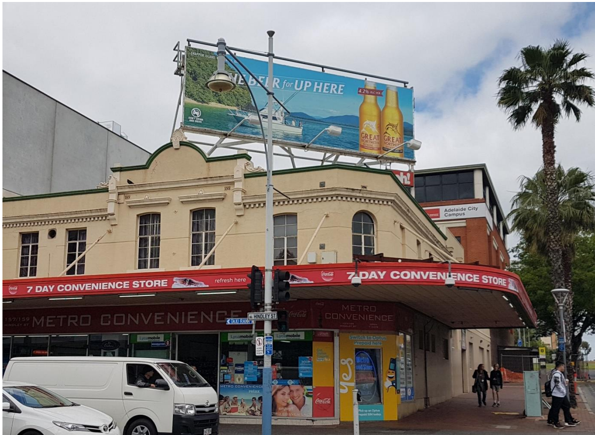
South east corner of same intersection roof sign displaying third party advertising
