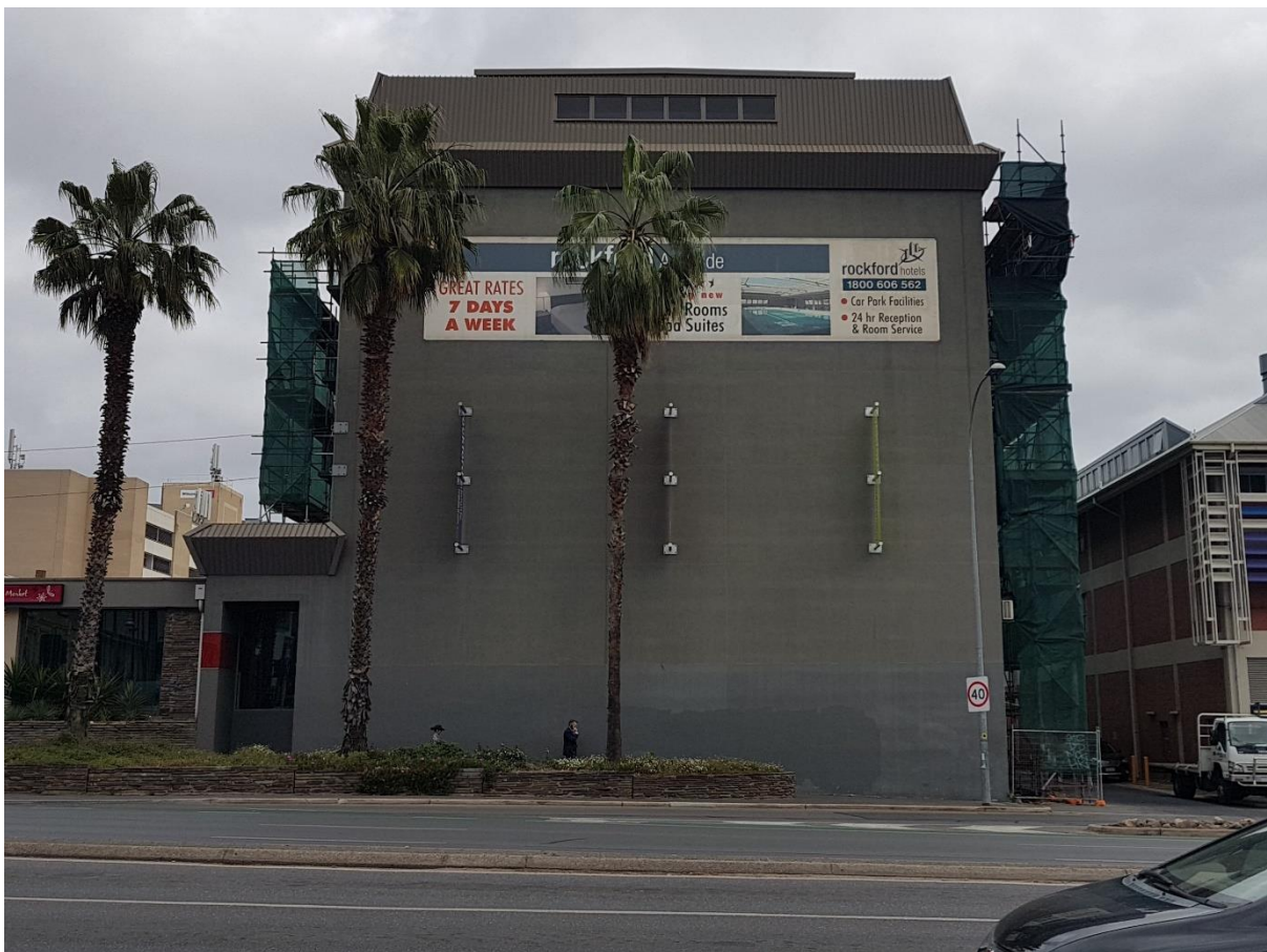
Existing eastern façade of Rockford Hotel located at 31-39 Morphett Street
